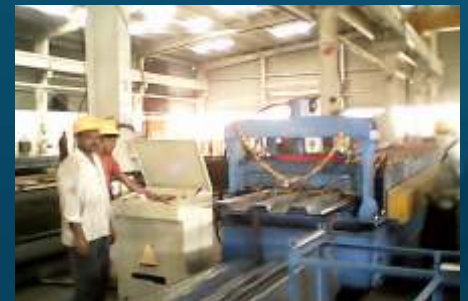
Decking Sheet Forming
